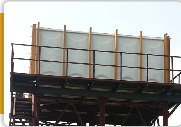
Diwana Railway Station
