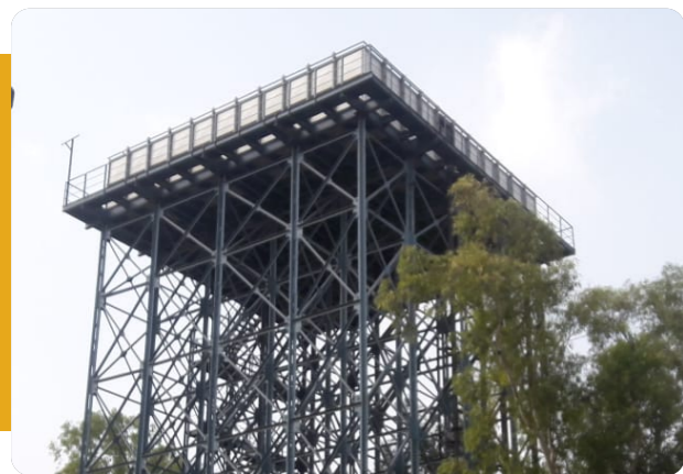
SMC Tank of 242KL (Shakurbasti Railway Station)
